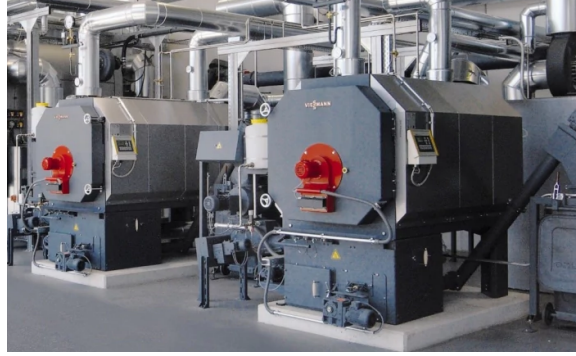
Figure 6. Viessman’s Vitoflex boilers, sized ~2.15 MMBtu heat input and below.
